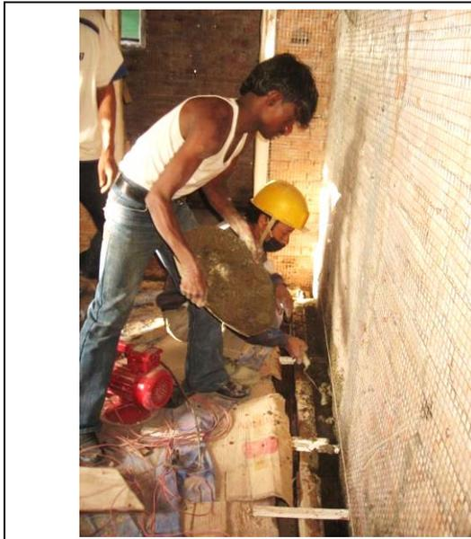
*Fig 5: GI wire mesh jacketing*
